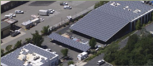
Our Headquarters, Auburn, CA 237 kW
